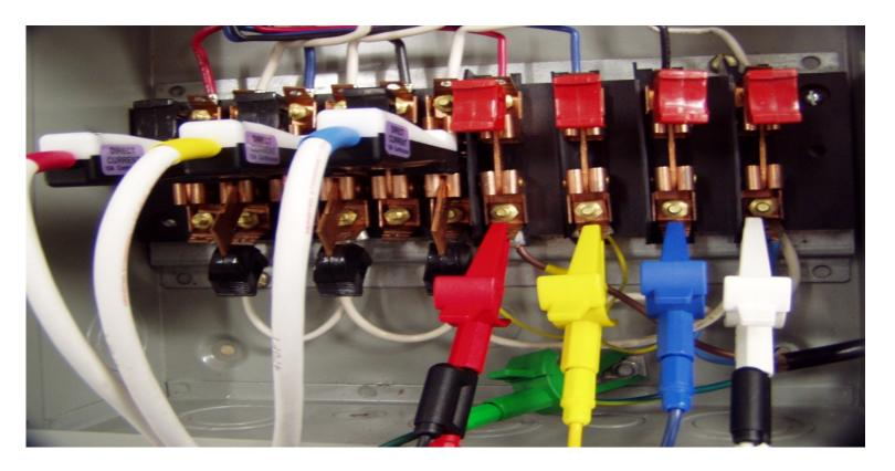
Current Connections Duckbill Connectors Voltage Connection Alligator Connectors
