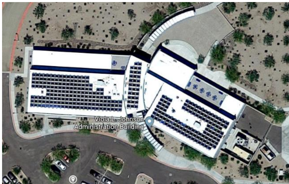
87kW Solar Farm at Hu Hu Kam Hospital Sacaton, AZ
